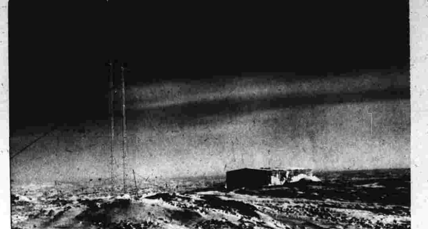
The "shack" in which Peter Brattis lived for over a year at the pole. It is one of the few buildings found above ground there, and had to be on the surface because Brattis' data-gathering equipment was inside, measuring the cosmic ray activity on the icy face of the polar area. The steel poles on the left support telephone lines which lead from the "shack" to the main barracks.
